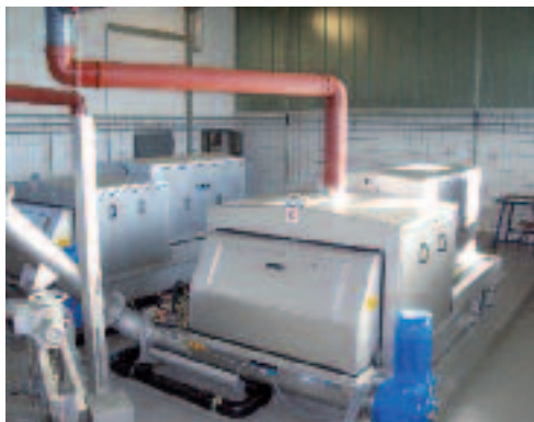
紧凑型CurveMax®弧型栅，进行可靠污水过滤
